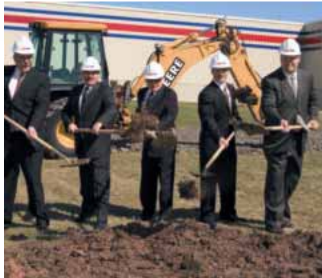
L-R: Vice President of Finance John Hosler, Executive Vice President and General Manager Dean Alexander, President and CEO Al Amatzio, Vice President and COO Alan Amatzio and Vice President of Operations Scott Davis break ground on the AMOIL Center expansion project.
