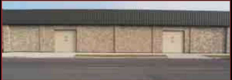
The most recent addition to the AMSOIL corporate headquarters is located just behind the main AMSOIL building. Complete renovation work inside and out began immediately upon acquisition. The structure was reinforced with all new steel beams, while a new roof, metal siding, commercial-sized automatic overhead doors and a handsome new stonework front capture the crafted décor of the other AMSOIL buildings.
